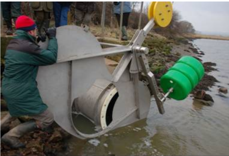
Figure 10. Tidal flap gate 1.4.2.2 Water quality and chemical barriers
