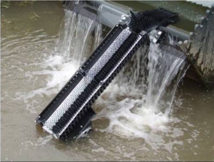
Figure 9. Bristle pass designed for a tilting weir
