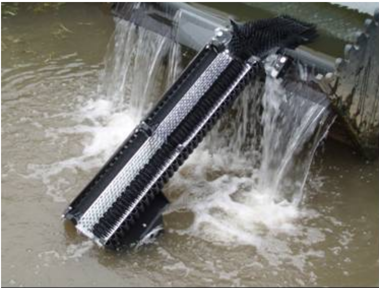
Figure 9. Bristle pass designed for a tilting weir
