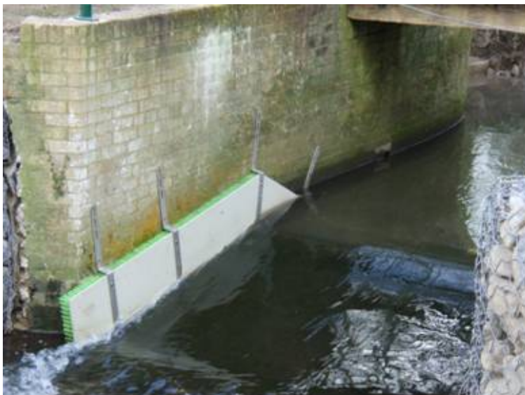
Figure 8. Bristle board eel pass
